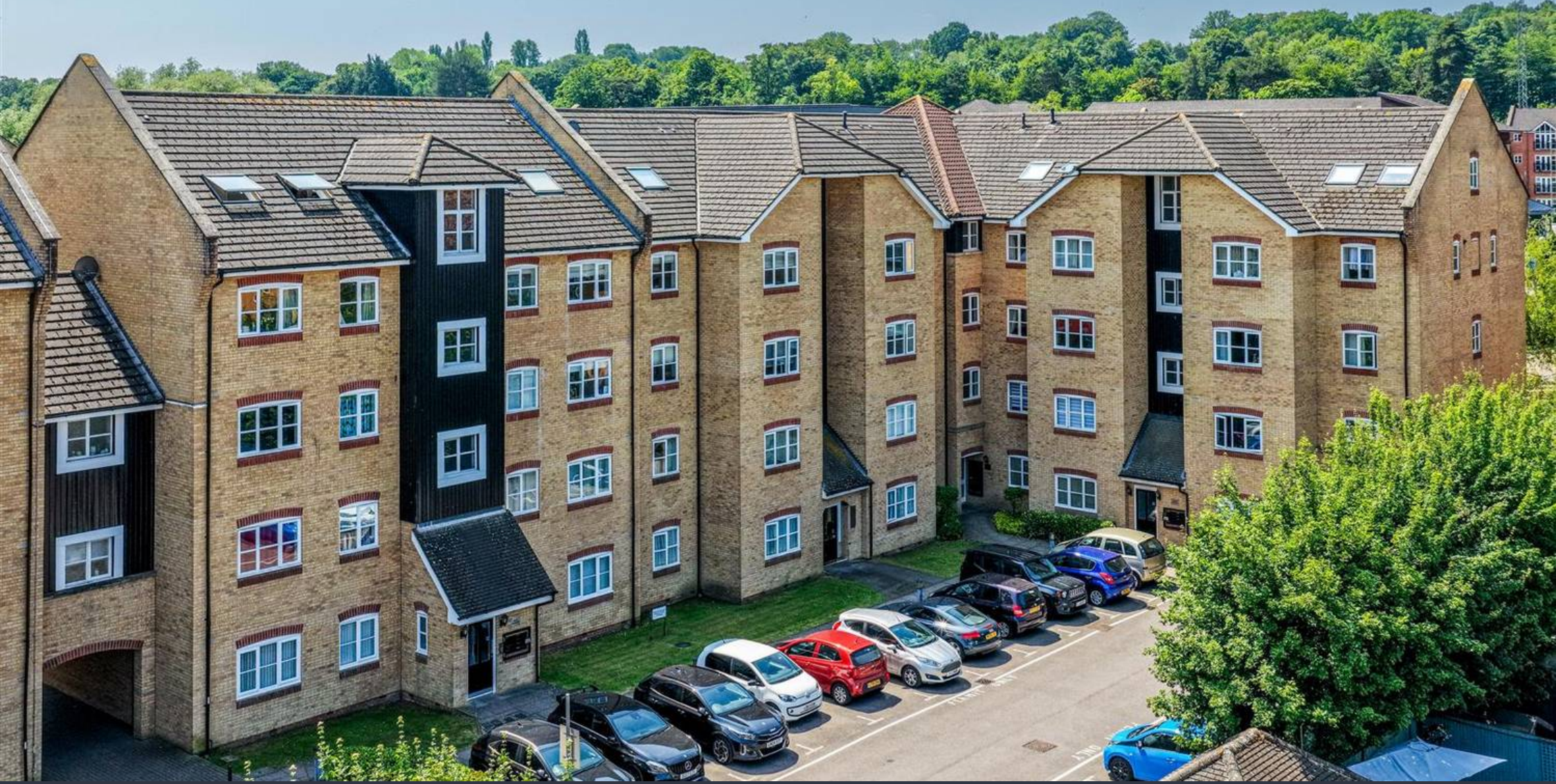
Evans Wharf, Hemel Hempstead £335,000
