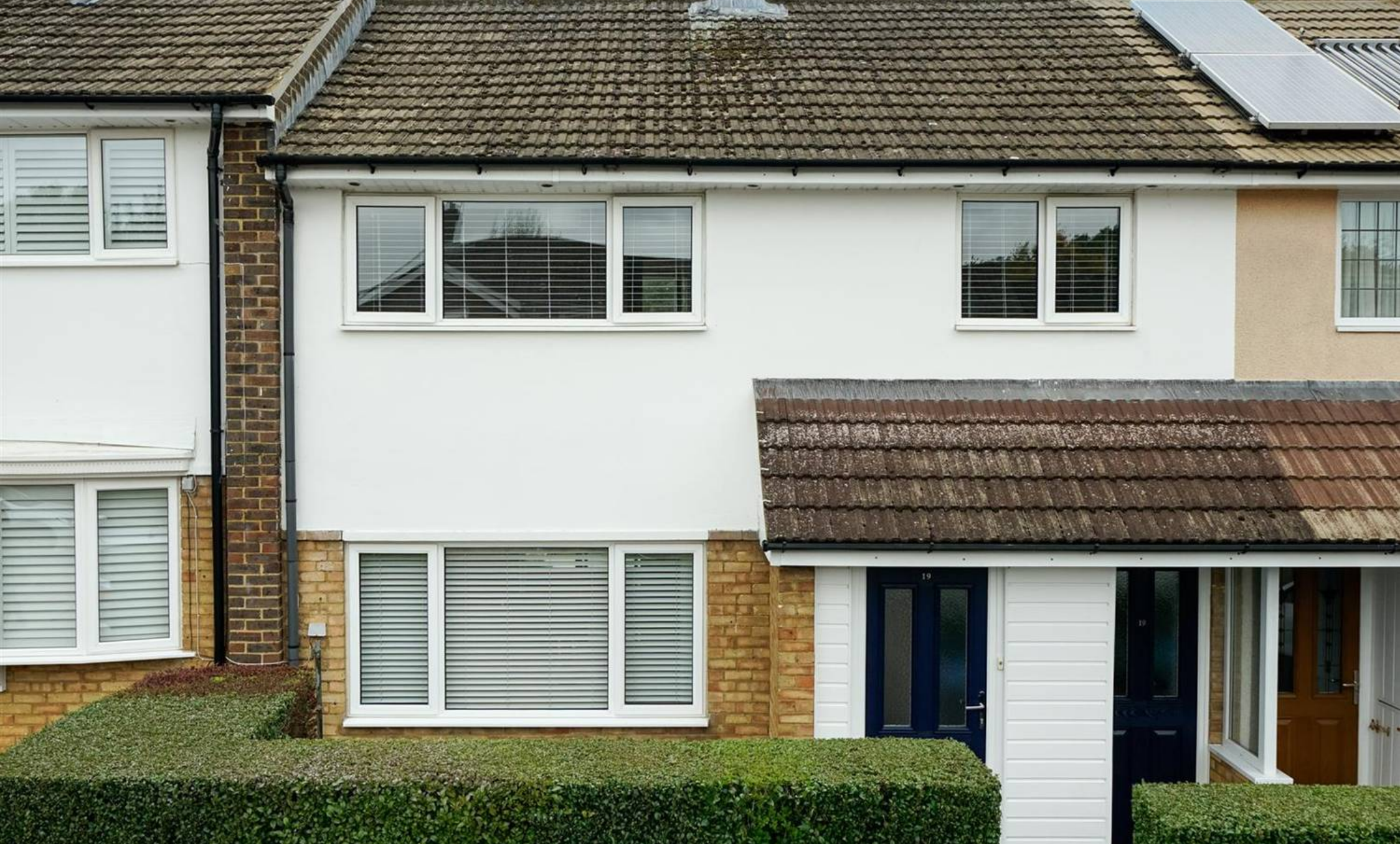
Gade Close, Hemel Hempstead
